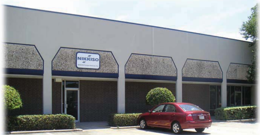
New NIKKISO Pumps America, Inc. US Headquarters in Houston, Texas. This new facility will support both Nikkiso's Metering Pump and Non-Seal Canned Motor Pump lines.
